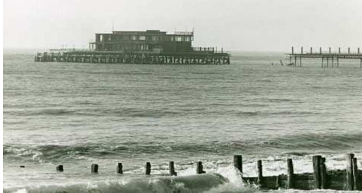
1940 – A section of the Pier was blown away by the military
