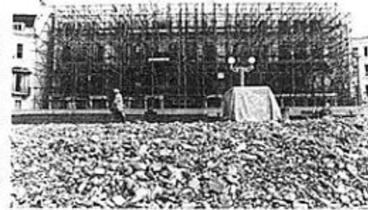
THE WARNES HOTEL masked by a mass of scaffolding.
